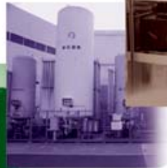
ON SITE PLANT
